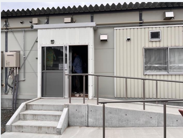
Entrance to a temporary housing in Rikuzentakata; stairs and elevation for wheelchairs were added later.
